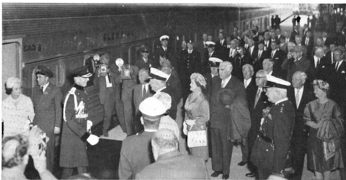
Scene at Spencer Street on arrival of the first standard gauge passenger train on 13th April, 1962.
