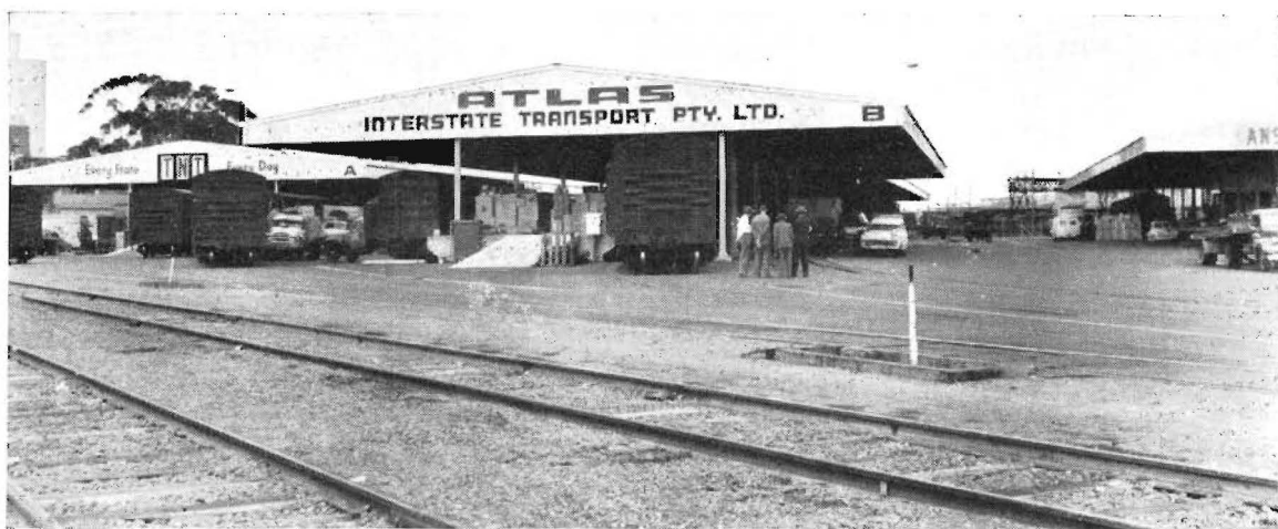
A section of the Forwarding Agents' Depot at North Dynon.
